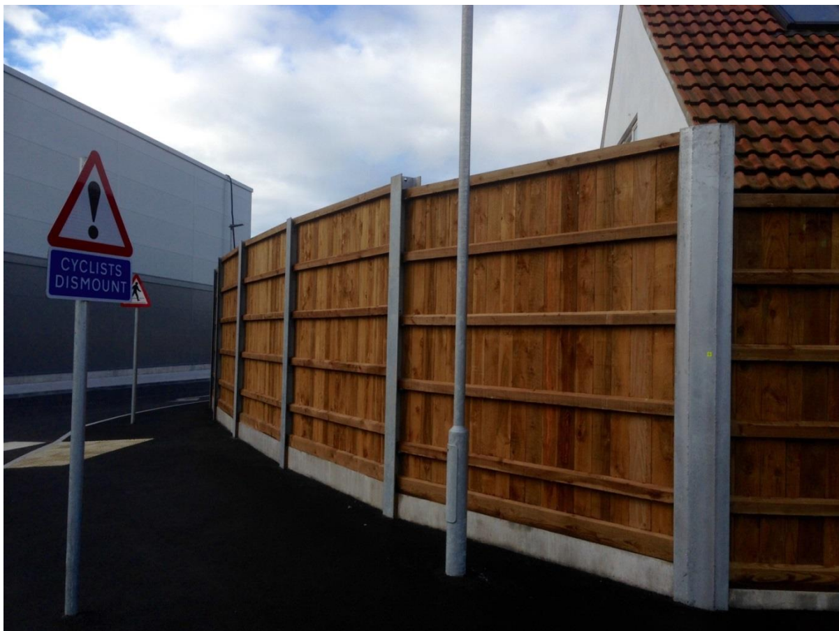
Photograph 4: An example of sound proof fencing.
